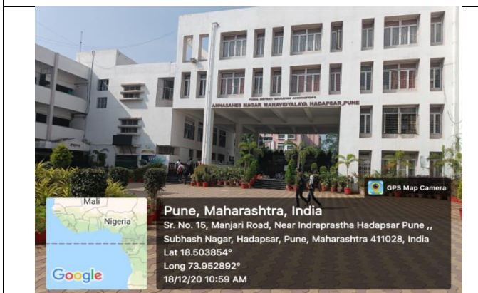
Shivaji Hall Building
